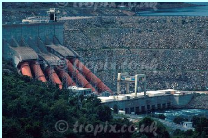
Electricity generating station at base of dam wall; huge pipes carry water past it from Lake Volta. Akasombo Dam, Ghana
